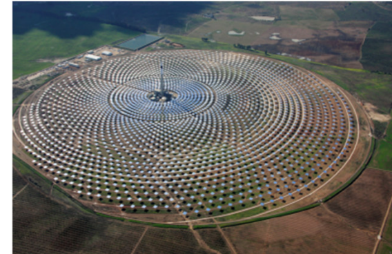
Gemasolar plant. Achieved 75 % Capacity factor with molten salt in first year of operation
