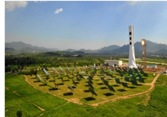
Beijing Badaling Solar Tower Once Through Direct Superheat Steam Generate
